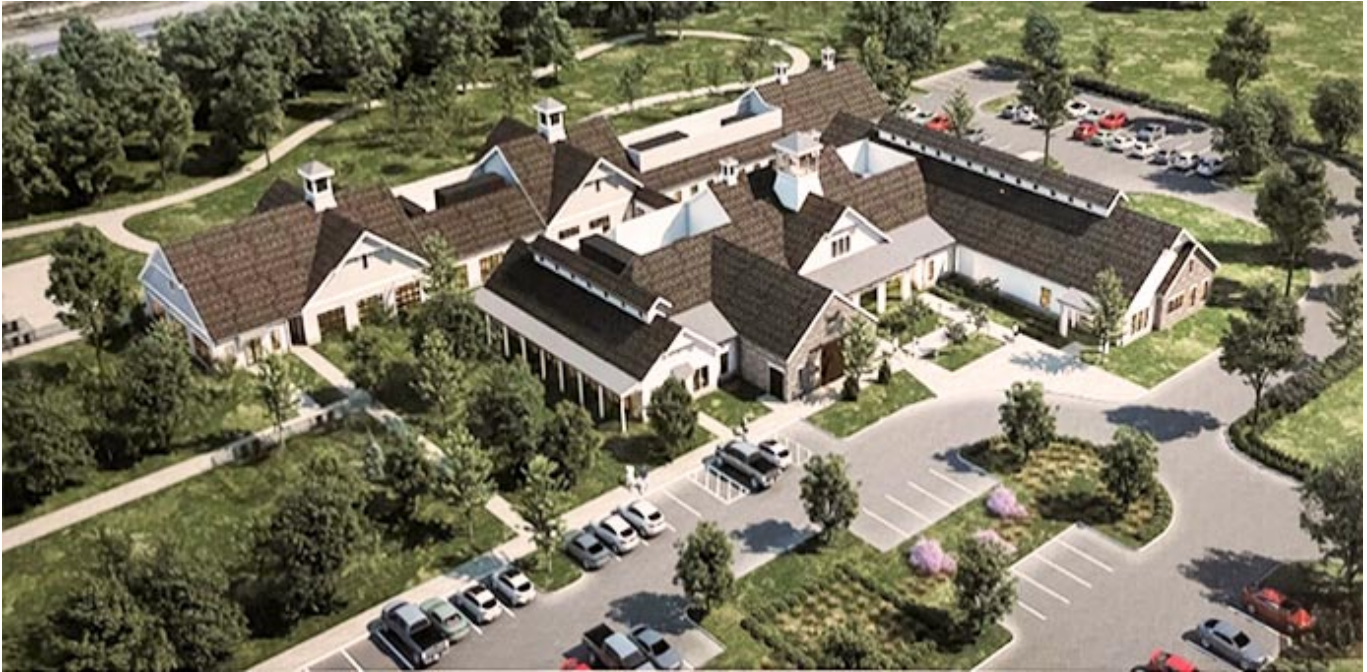
Williamson County Animal Center expansion project
