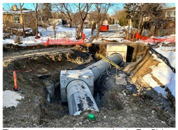
The storm sewer newly connected to the Toe Blake Park collector, which was the source of the St. Pierre River. The riverbed, which can be seen in the bottom right of the picture, no longer has any flow as all the river water is now being bypassed through the storm sewer which will soon be completely buried.
