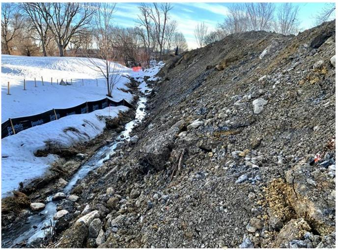
This picture shows the small amount of frozen water remaining in the St. Pierre riverbed. A large pile of rocks and soil from the digging of the trench for the storm sewer looms over the river. Thankfully City workers assured that the riverbed would not be filled in and that all soil not used to bury the sewer would be removed.
