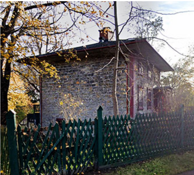
Side of the Goode house as seen from Cote St. Antoine Road – Image: Google Maps
