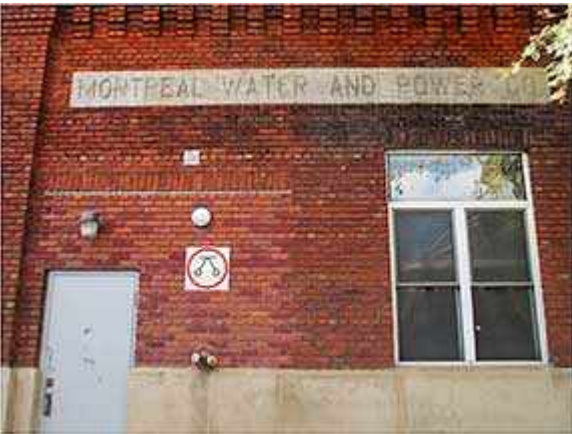
Former Montreal Water & Power Company (1930) building on
